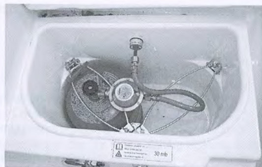
Gas bottle with 30 mbar pressure relief valve
