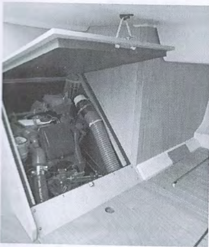
Access engine compartment (1)
